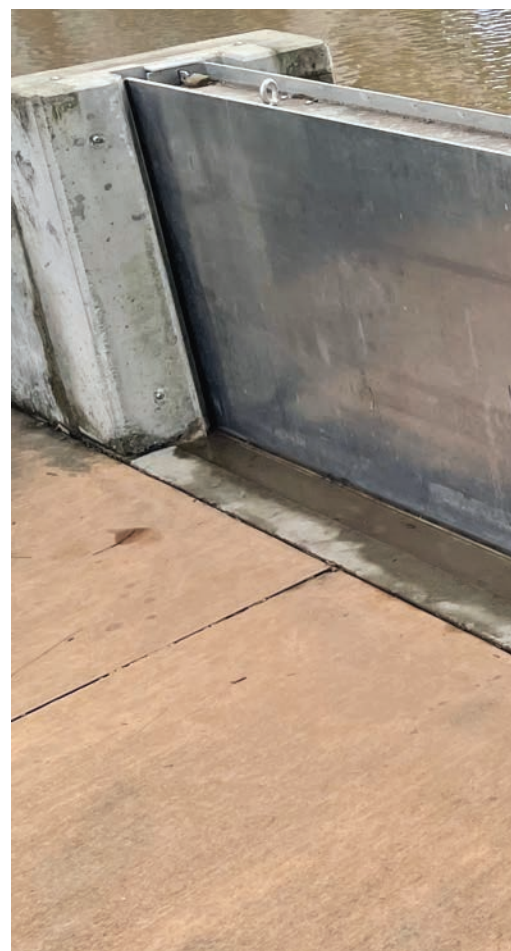
Figure 6: Example of a retractable flood barrier protecting community assets
