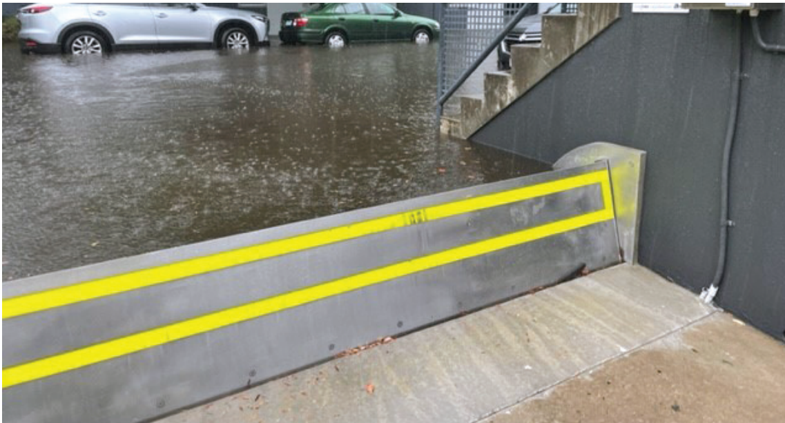
Figure 13: Example of a buoyant tilting flood barrier
