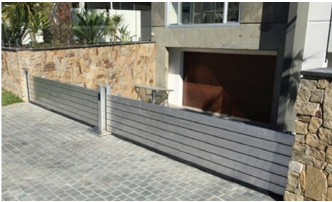
Figure 9: Example of a temporary demountable flood barrier protecting critical infrastructure
