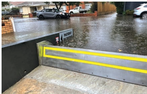
Figure 3: Examples of buoyant (or passive) flood barriers
