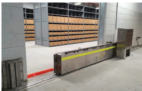
Figure 4: Examples of actuated flood barriers
