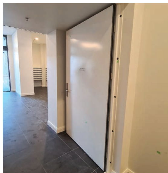
Figure 12: Example of a permanent manual flood barrier door
