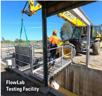
Installing Screen Retrieval Systems
