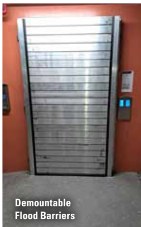
Demountable Bulkhead Flood Barriers
