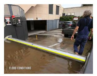
^ Pictured above is the FloodFree Passive Tilting Flood Barrier which self-deploys as water levels rise.
