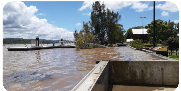
The Maclean waterfront precinct in flood, featuring deployed AWMA FloodFree Retractable Barriers.
