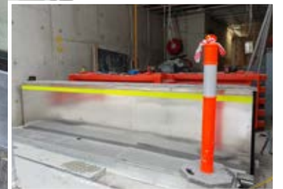
Left- Completed Concealed Flood Barrier Right- Concealed Flood Barrier during installation
